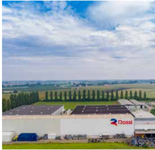
High precision manufacturing facility Ganaceto (Modena) - Italy
